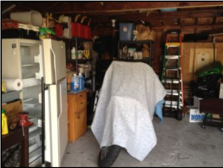
some portions of the garage were not viewable due to item storage
